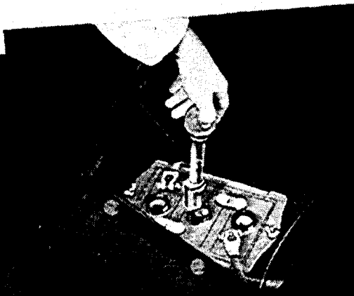
READILY ACCESSIBLE BATTERY
