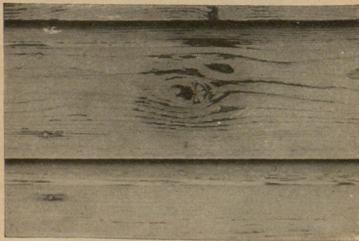
FIGURE 20.— Failure of paint over a knot that had been shellacked prior to painting.
