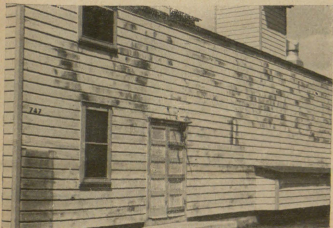
FIGURE 10.— Typical discoloration of paint due to mildew. Before repainting, surface should be scrubbed with water containing some alkaline cleaner, for example, trisodium phosphate.
